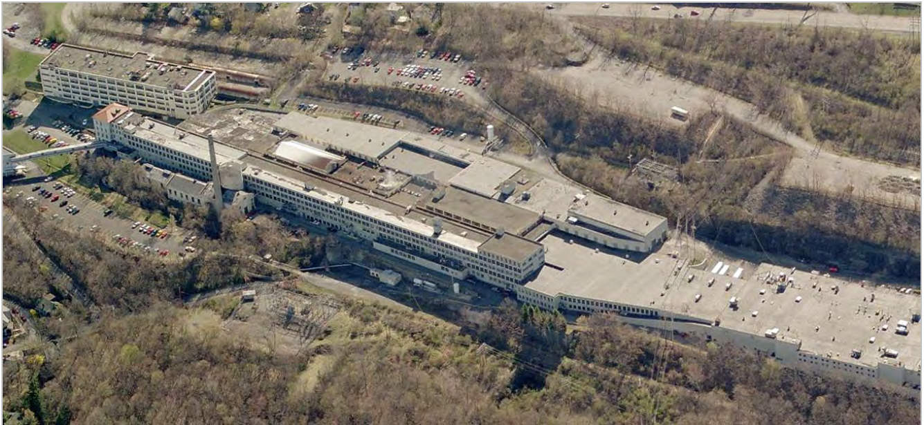
Emerson Power Transmission Facility (Pictometry)
