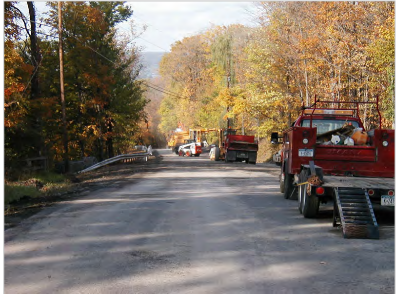
Maintenance activity on Stone Quarry Road.
