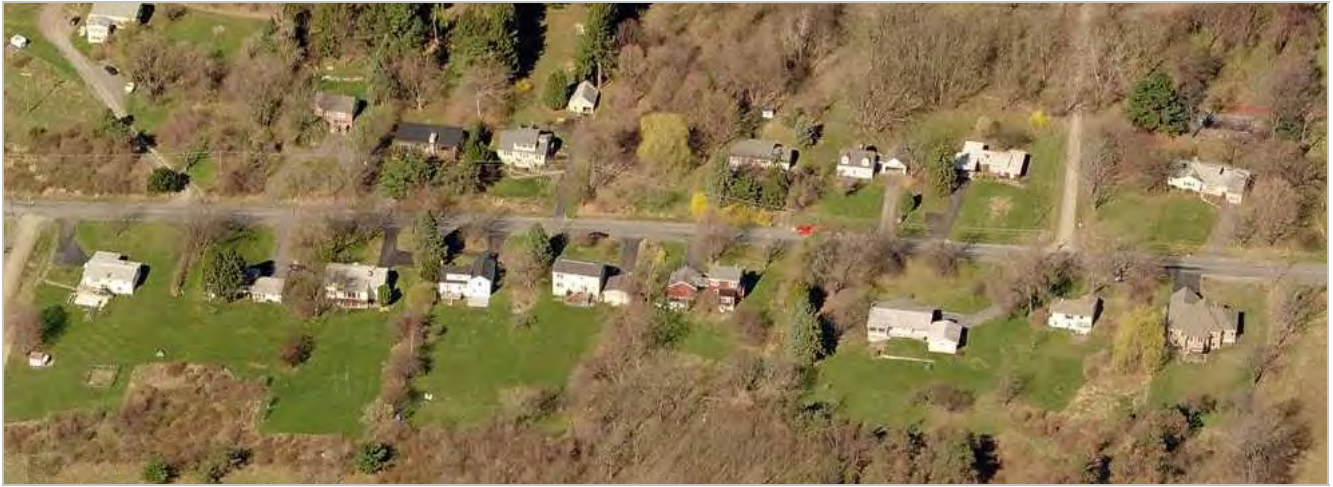
Frontage development, Westhaven Road, West Hill area. (Pictometry)
