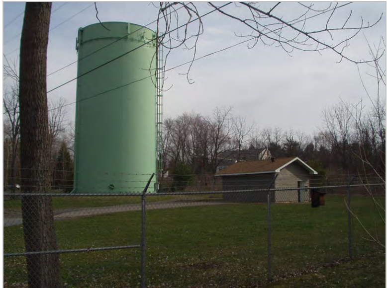
Christopher Circle water tank.
