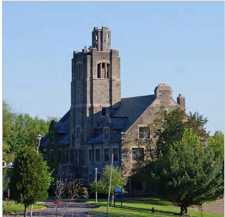
Former Grand Lodge of the International Order of Odd Fellows/Rebekah's Home, located on Trumansburg Road
