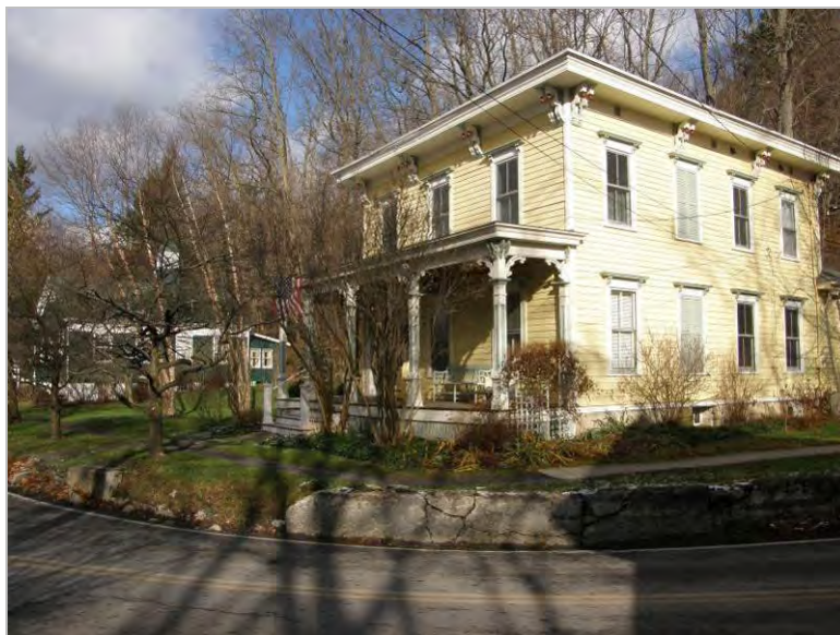
House in Forest Home neighborhood
