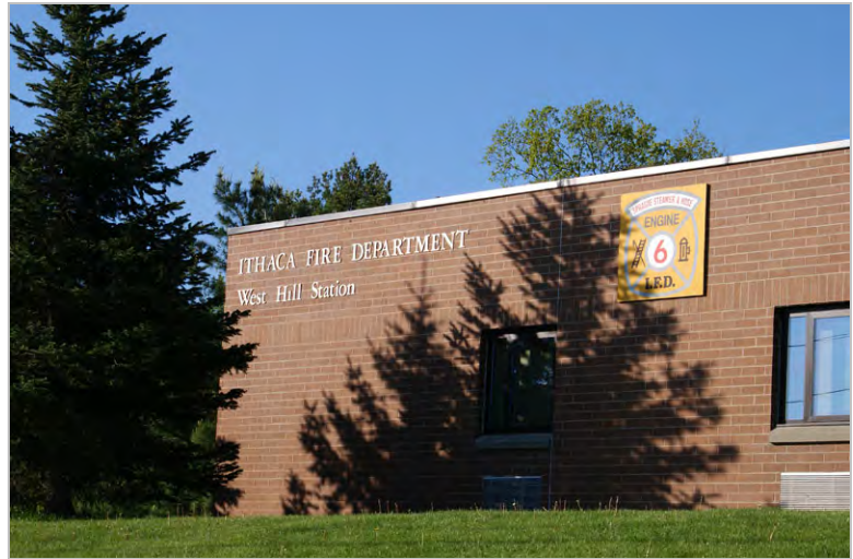
IFD West Hill Station on Trumansburg Road.
